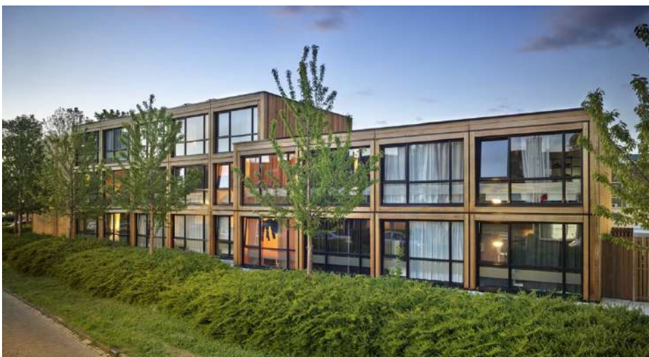
Figure 20: 38 prefabricated homes in Alkmaar (picture by: Finch Buildings, 2020)
